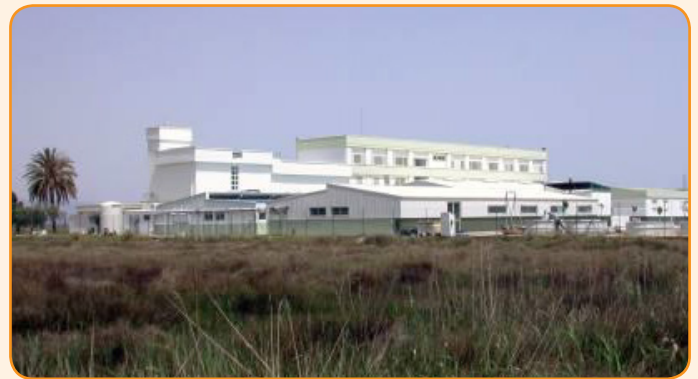
View of the 4 buildings (A-D) which compose installation IATS-EXP within the campus of the Instituto de Acuicultura Torre de la Sal.
